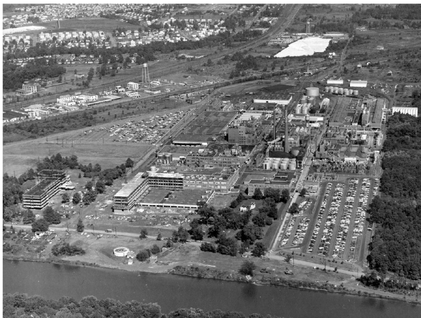
Figure 10. High water mark for the Bakelite plant 1957. Two R&D buildings under construction at lower left. Facing East. Plant employee parking lots (right front, left rear) are full. But Suburbia is approaching from North. Courtesy of the Leo Hendrik Baekeland Award Collection, North Jersey Section of the American Chemical Society.
