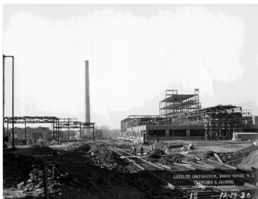
Plant about to open while construction continues (Winter 1930/31).
